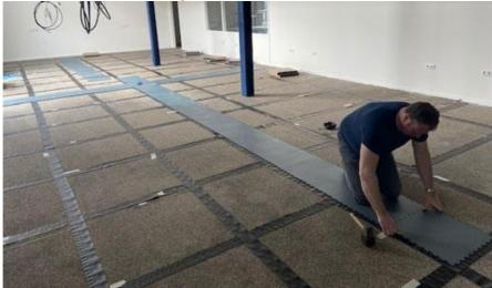
6- First copy the X and Y axis by a line of tiles, this will give you a properly outlined and parallel lay-out:
