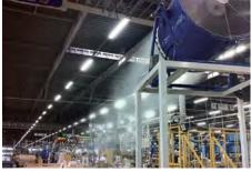
Cooling system with COOLJetter®, providing effective and low-cost cooling for large spaces.
